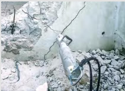
Demolition of concrete and reinforced concrete
