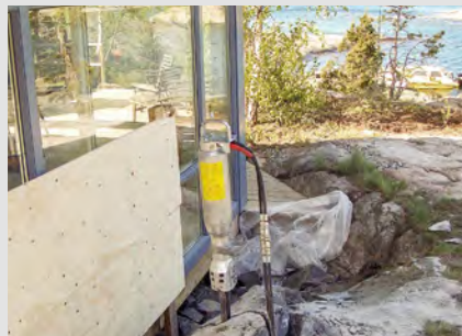
Demolition of rock and natural stone
