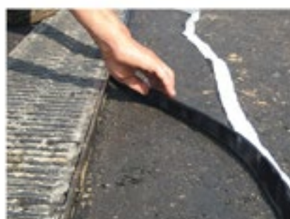
TOK®-Band SK used on drainage channels in asphalt surfaces.
